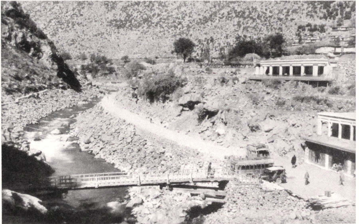
Fig. 48 - Bahrein. Bridge on the Swat River.
